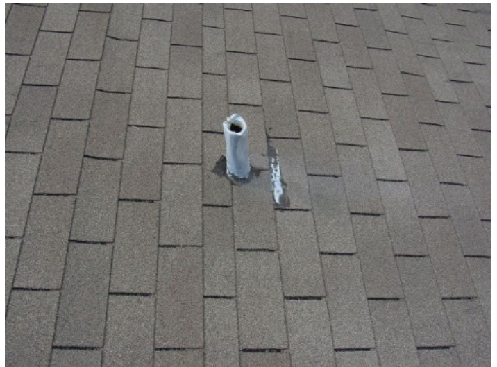
Roof penetrations looked good
