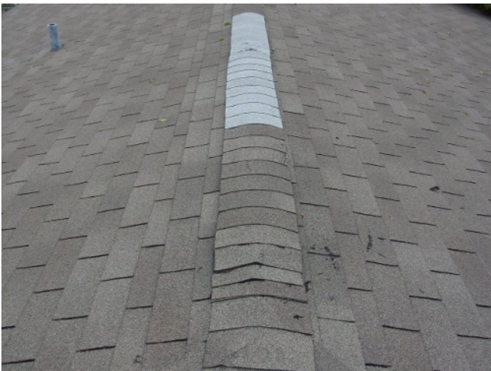
Ridge vent - some shingles replaced
