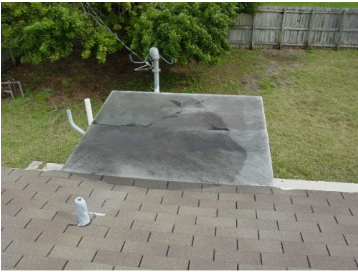
Flat roof over the utility room looked good
